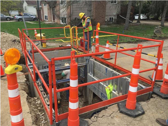
**Atmospheric testing should be necessary when trenching projects involve work in and around sewers, gas utility systems, landfills, refineries, chemical plants or hazardous waste dumps.**
