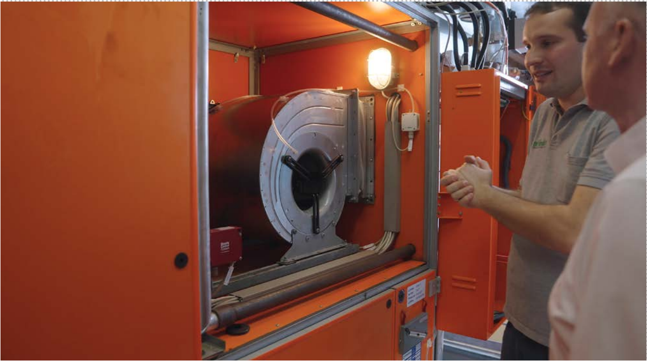
FIGURE 4: Thanks to EC motors, the new RadiFit is much more economical and could be replaced quickly and easily.
