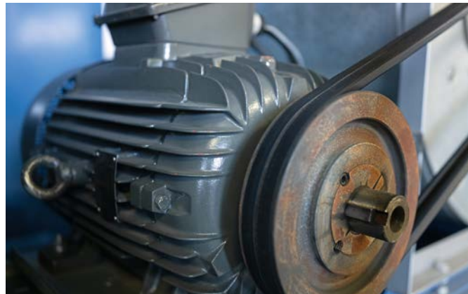
FIGURE 3A + B: The large belt-driven centrifugal fans for supply and exhaust air were inefficient, loud, and already corroded.
