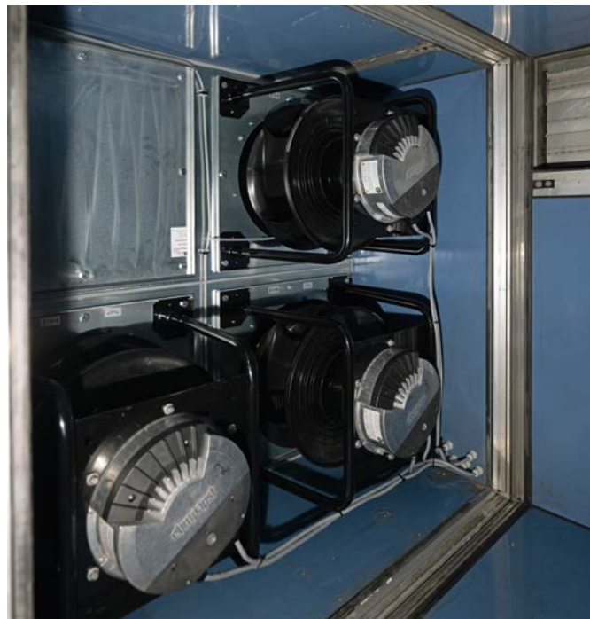
FIGURE 4: The old fans were replaced with a FanGrid with three centrifugal fans from the latest RadiPac generation.
